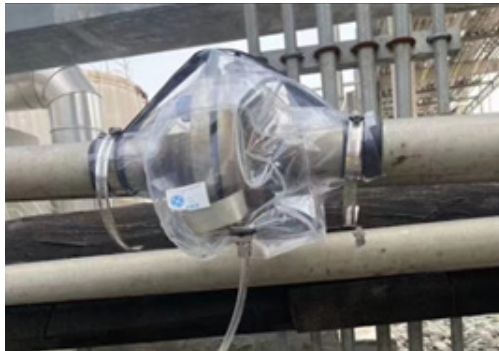
Flange Shield fitted with PTFE Drain
